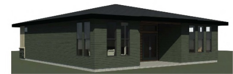
HIP ROOF - BACK VIEW
